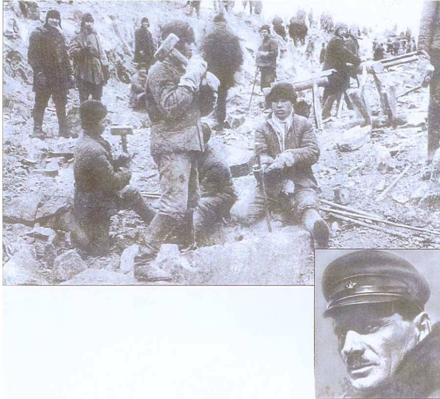
Instead of dynamite, prisoners broke up the large boulders using hammers and iron rods. Inset: Naftaly Frenkel
