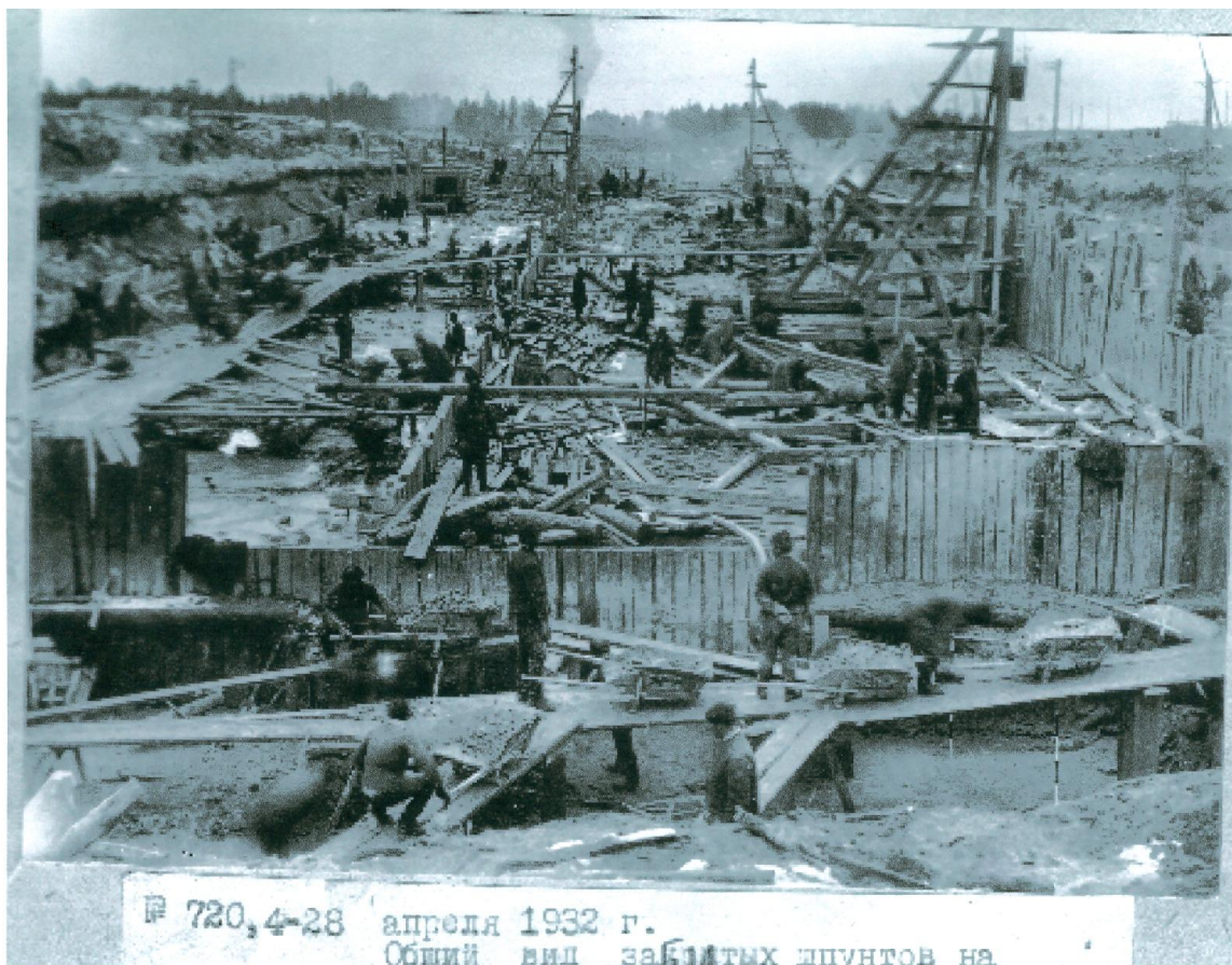
The route was divided into nine sections. Everywhere there were platforms, scaffolding, wooden derricks, nets, ropes, pulleys and hoists to make the work easier.
