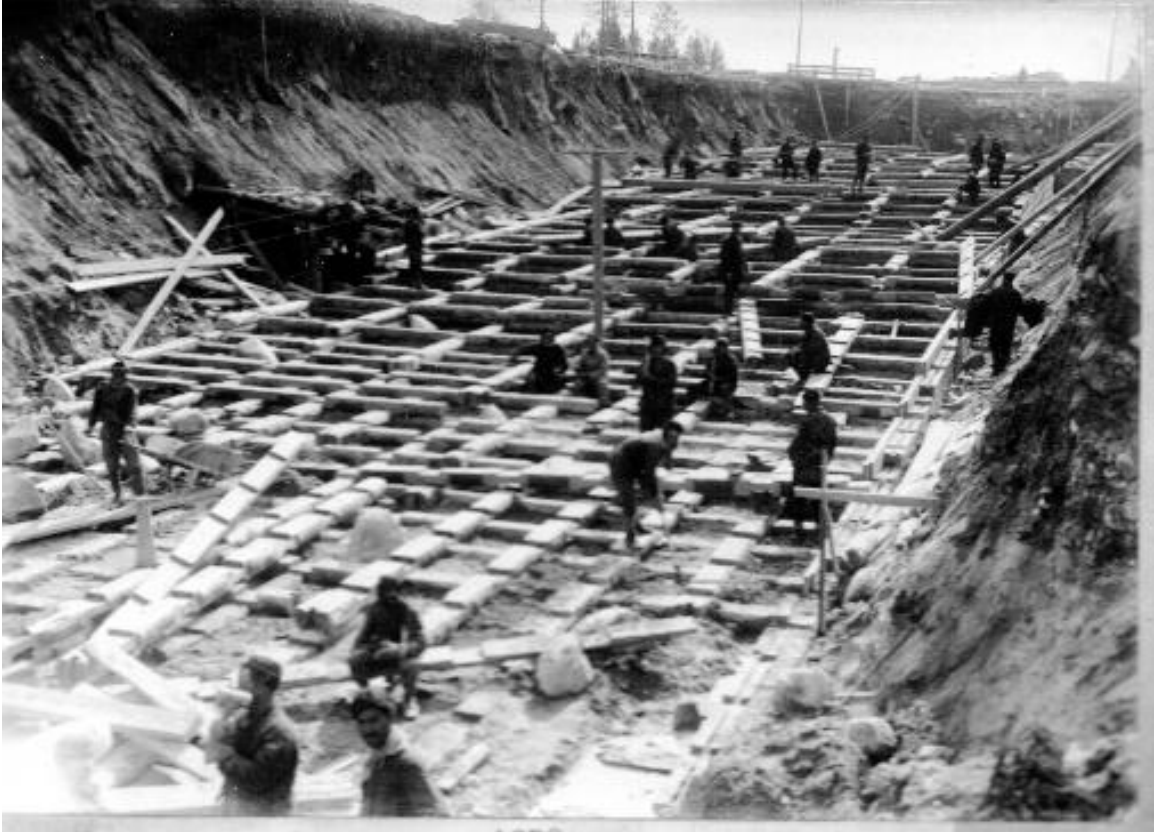
The walls of the locks were built with logs, fitted and joined together as cribs, then erected and filled with dirt and stones.
