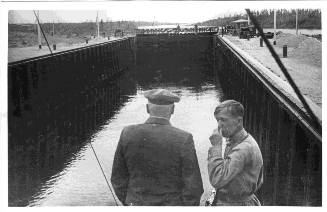
Final inspections were made by the engineers to assure that the work was done properly.
