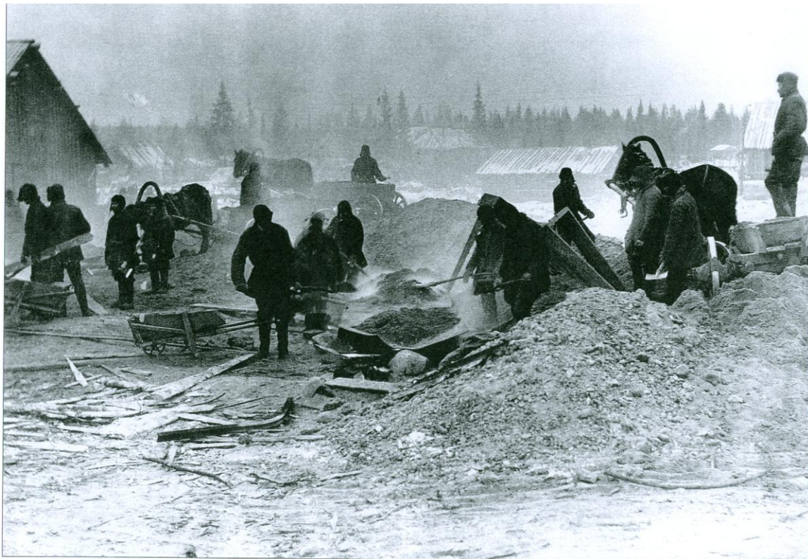
Prisoners also had to heat mortar to help it bond in freezing weather.
