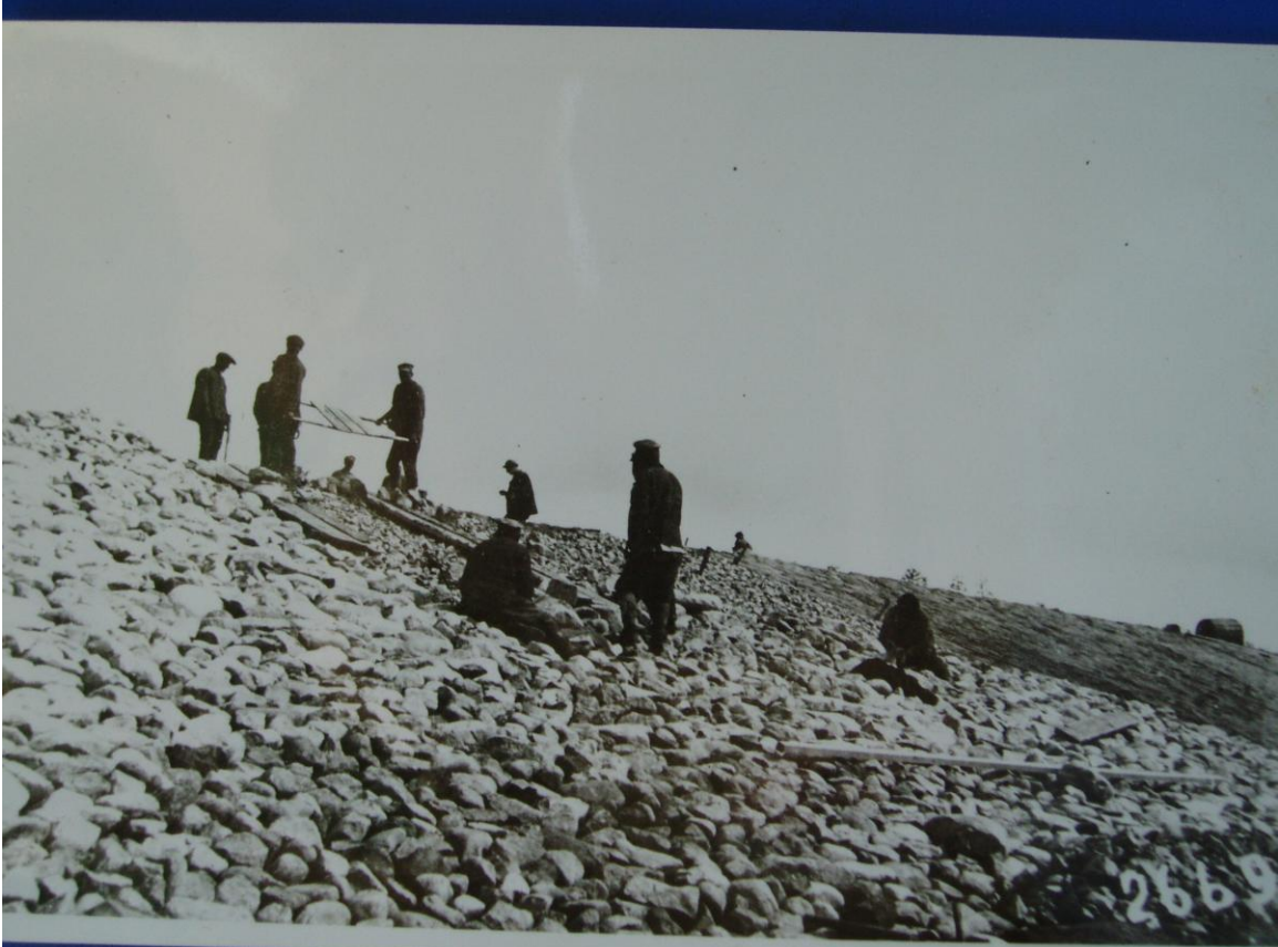
The many stones needed to line the canal banks were all carried by hand.
